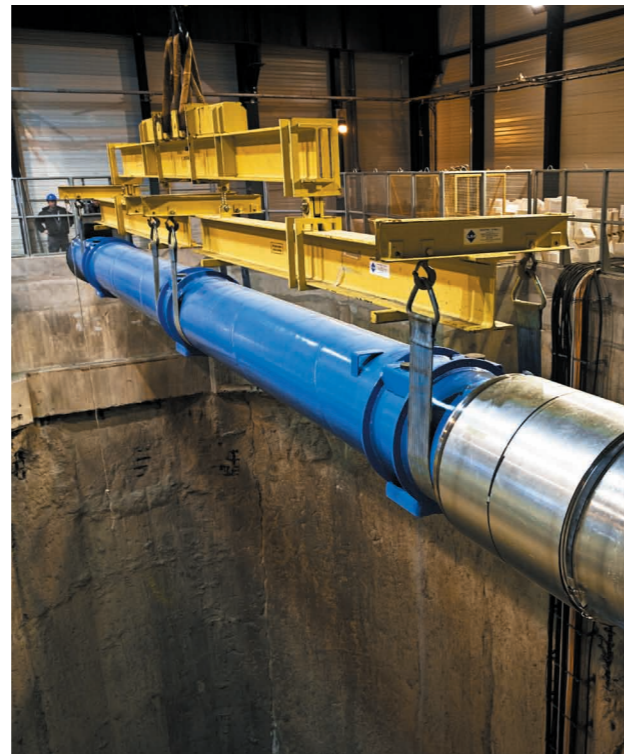
A replacement magnet for LHC sector 3-4 being lowered in the tunnel
